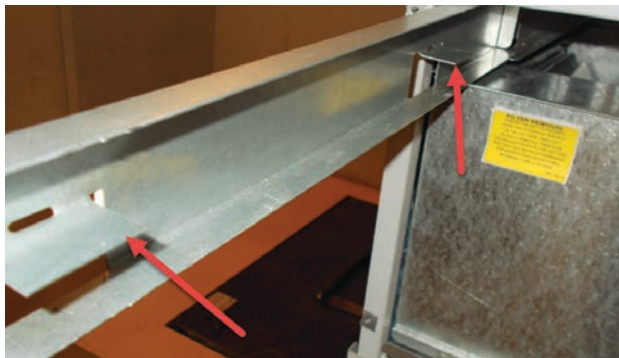
FIGURE 4 Filter Tabs in Up Position
