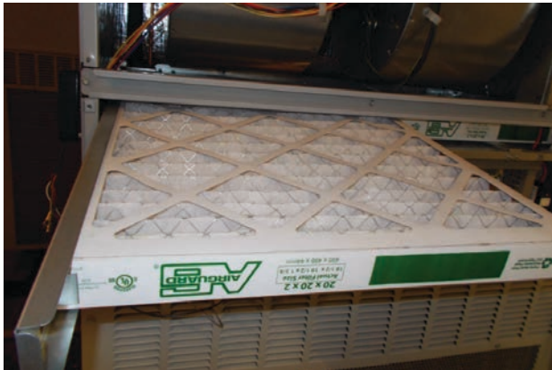
FIGURE 10 Install Left 2" Filter
