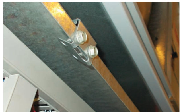
FIGURE 8 Re-Install Screws and Bend Tabs Up
