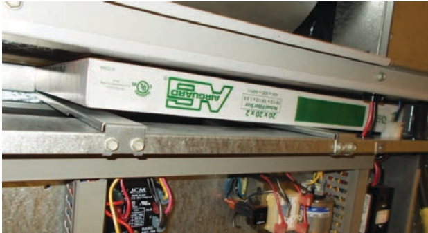
FIGURE 10 Install Left 2" Filter
