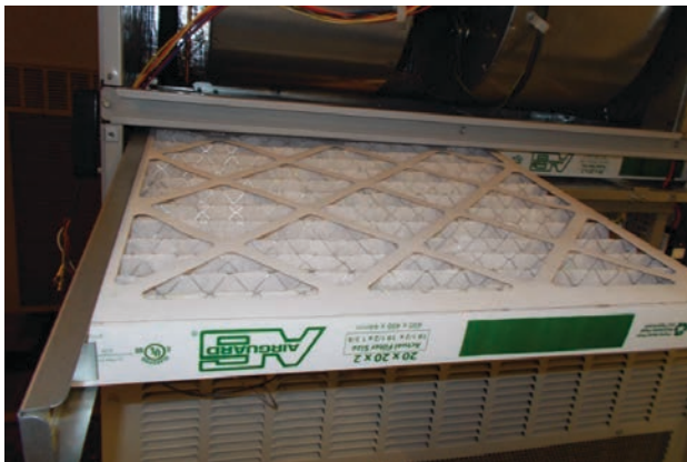
FIGURE 10 Install Left 2" Filter
