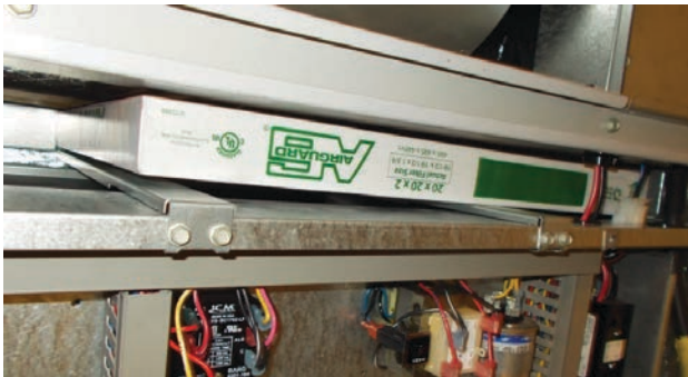
FIGURE 10 Install Left 2" Filter
