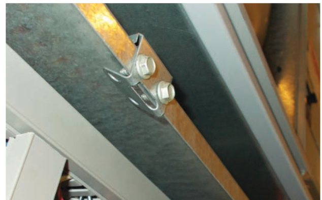
FIGURE 8 Re-Install Screws and Bend Tabs Up
