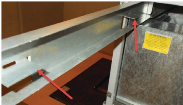
FIGURE 4 Filter Tabs in Up Position
