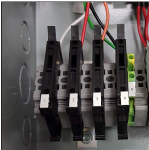
FIGURE 13 LC6000 Fused Power Supply Terminal
