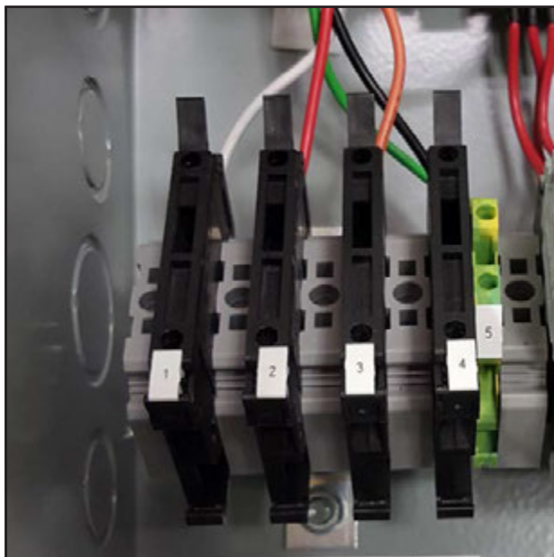
FIGURE 13 LC6000 Fused Power Supply Terminal
