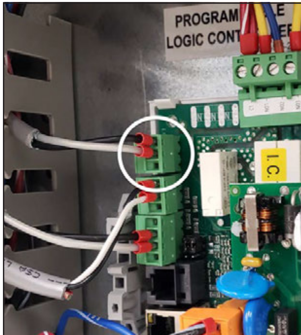
FIGURE 86 Expansion Module (c.pCOe) Communication Wires
