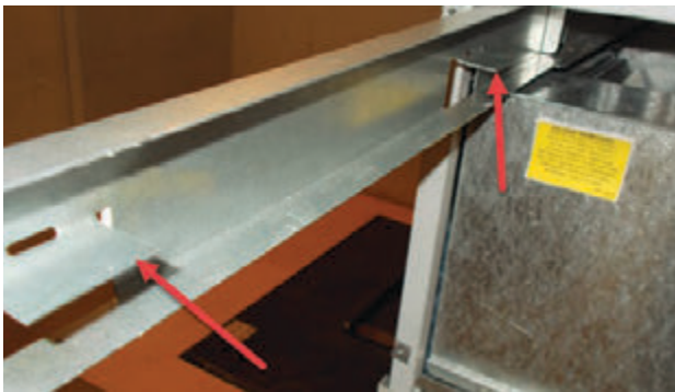
FIGURE 4 Filter Tabs in Up Position (1" Filter)
