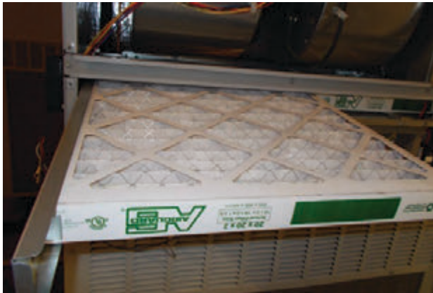
FIGURE 10 Install Left 2" Filter
