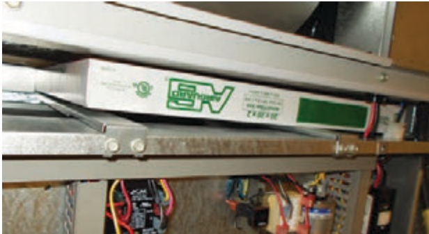
FIGURE 10 Install Left 2" Filter
