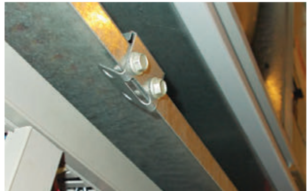
FIGURE 8 Re-Install Screws and Bend Tabs Up
