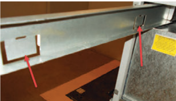
FIGURE 5 Bend Filter Tabs Down
