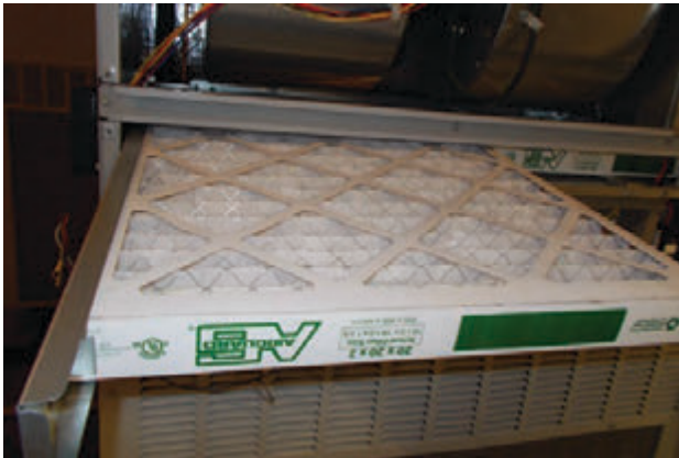
FIGURE 10 Install Left 2" Filter
