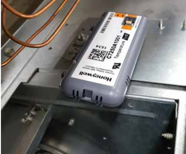
FIGURE 13 Mixed Air Temperature Sensor Location
