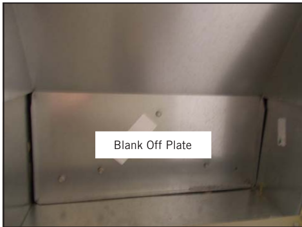
FIGURE 4 Remove Blank Off Plates (Both Sides)
