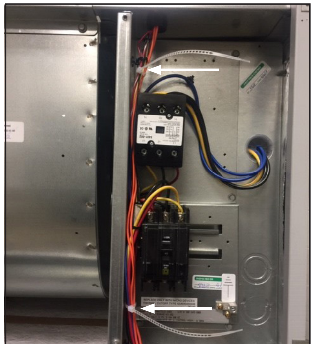
FIGURE 15 Secure Sensor Wires with Ladder Ties
