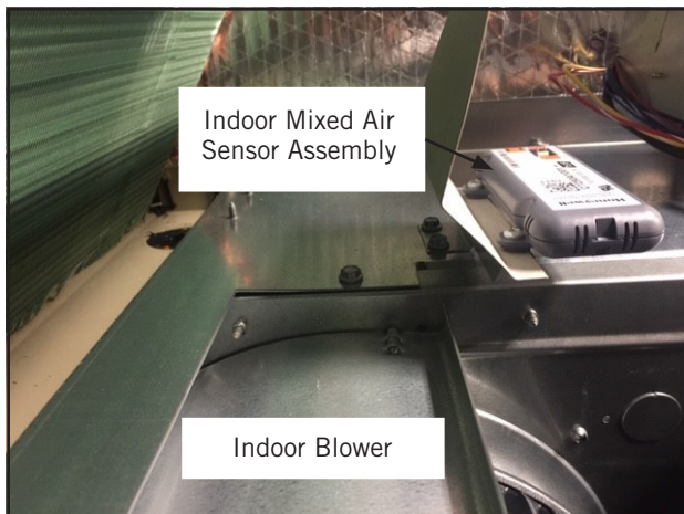
FIGURE 13 Install Indoor Mixed Air Sensor Assembly
