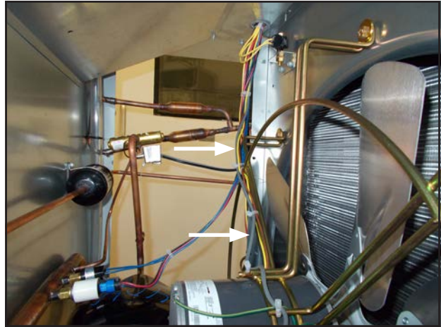
FIGURE 19 Route Wires and Secure with Ties
