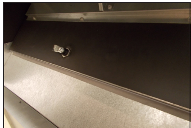
FIGURE 24 Exhaust Blade and Latch
