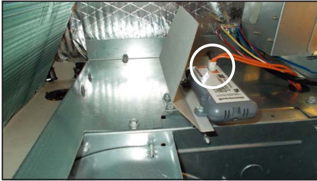
FIGURE 16 Connect Mixed Air Sensor Plug
