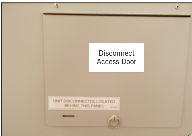
FIGURE 1 Disconnect Power
