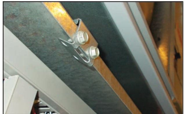
FIGURE 8 Re-Install Screws and Bend Tabs Up
