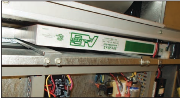
FIGURE 10 Install Left 2" Filter
