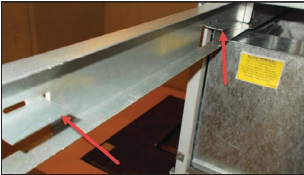
FIGURE 4 Filter Tabs in Up Position
