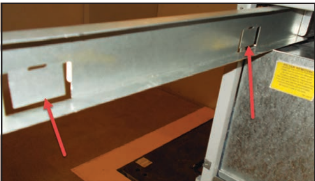
FIGURE 5 Bend Filter Tabs Down
