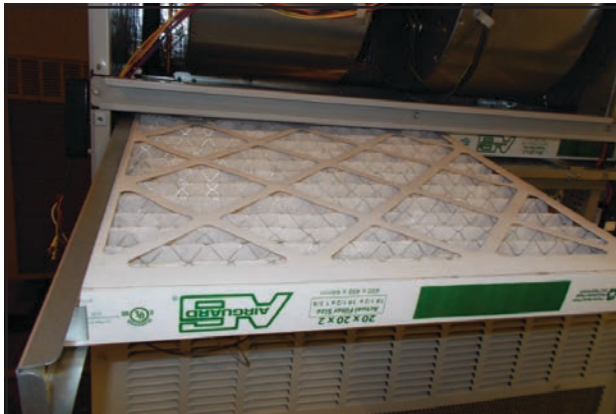
FIGURE 10 Install Left 2" Filter
