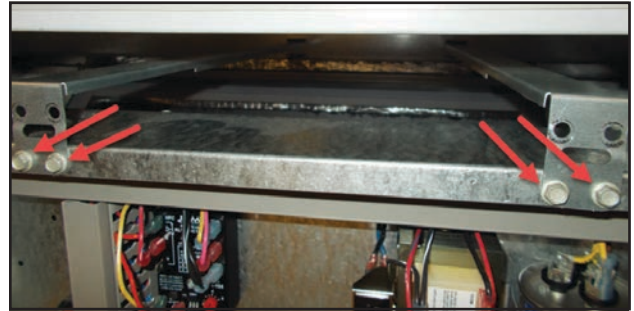
FIGURE 6 Remove Four Screws
