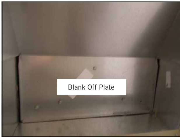
FIGURE 4 Remove Blank-Off Plates (Both Sides)
