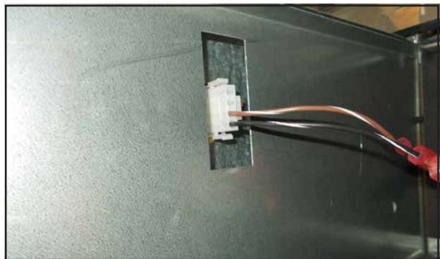
FIGURE 12 Connect CRV Power Plug to Control Panel Plug
