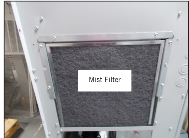
FIGURE 16 Install Mist Filters
