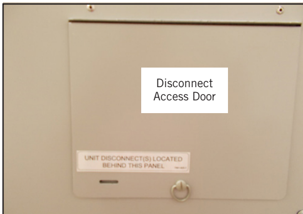
FIGURE 1 Disconnect Power
