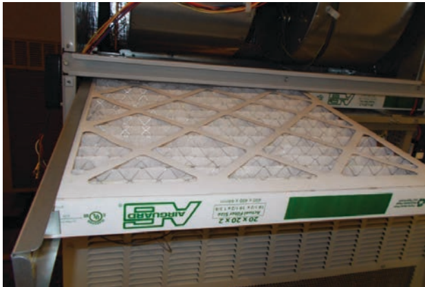
FIGURE 10 Install Left 2" Filter
