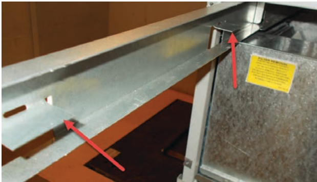
FIGURE 4 Filter Tabs in Up Position (1" Filter)
