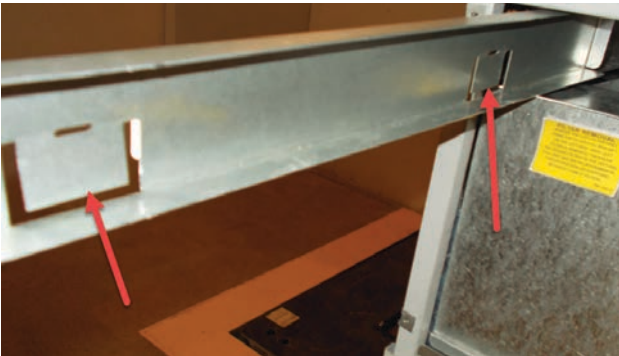
FIGURE 5 Bend Filter Tabs Down (2 inch Filter)
