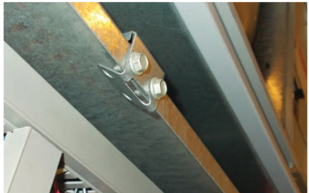
FIGURE 8 Re-Install Screws and Bend Tabs Up
