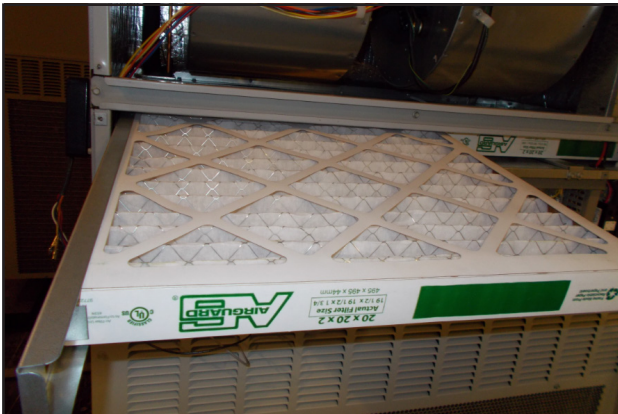
FIGURE 67 Install Left 2" Filter
