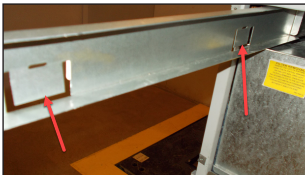
FIGURE 62 Bend Filter Tabs Down
