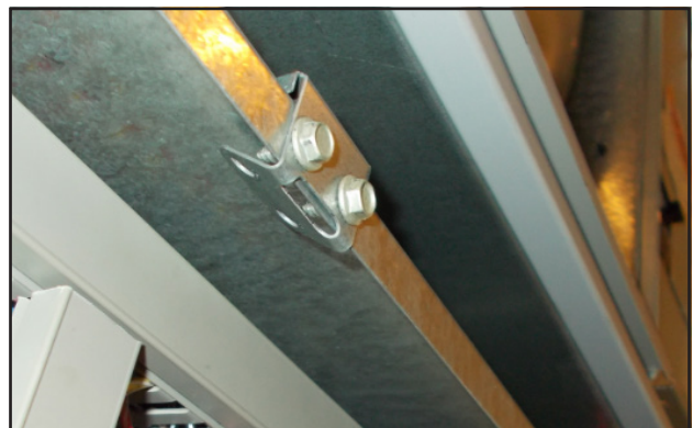
FIGURE 65 Re-Install Screws and Bend Tabs Up
