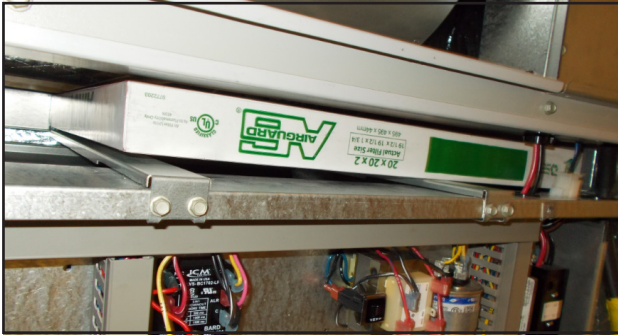
FIGURE 66 Install Right 2" Filter
