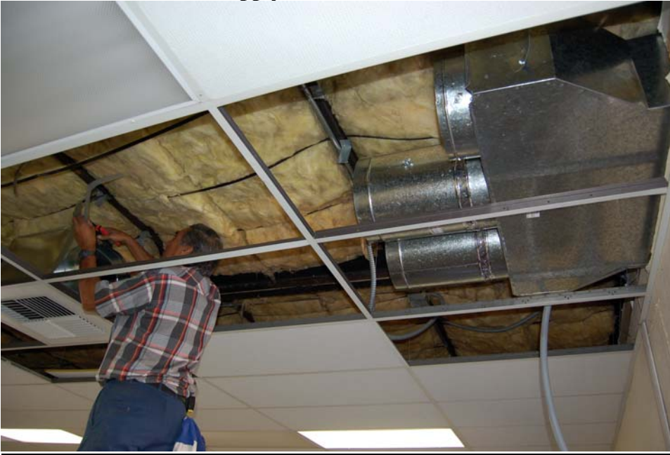
Installation of 3 outlet supply ducts
