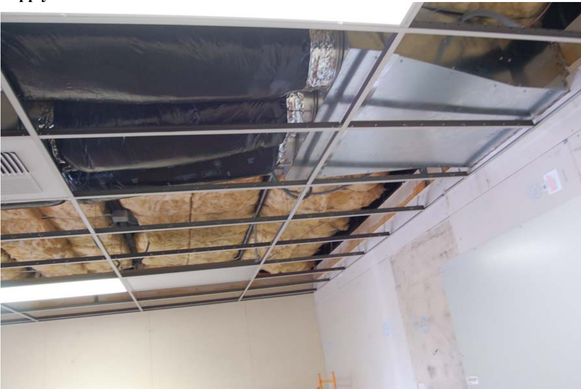
Supply Air Acoustical Plenum installed – 3 outlets.
