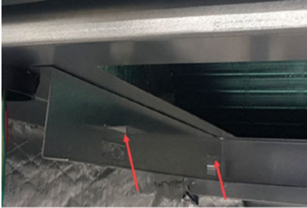
FIGURE 10 Bend Filter Tabs Down
