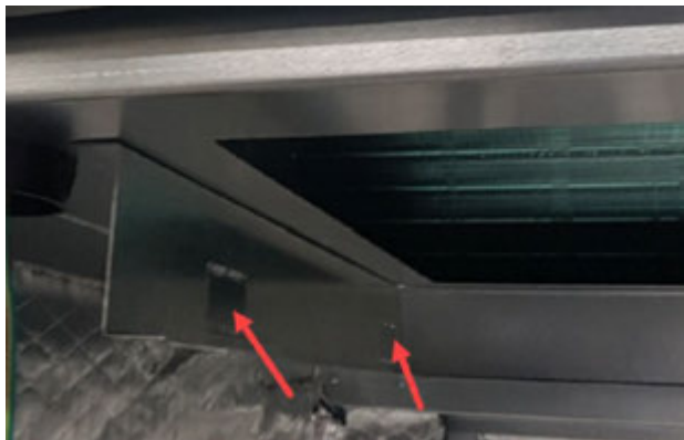
FIGURE 10 Bend Filter Tabs Down
