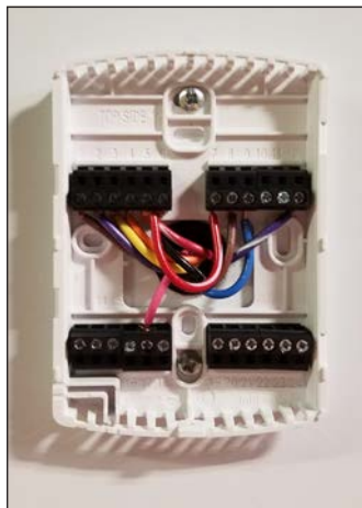
FIGURE 4 Connect Wires to Thermostat Sub-Base
