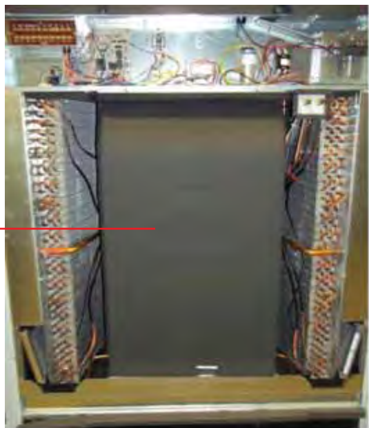
FIGURE 4 REMOVAL OF AIR DUCT
