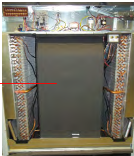
FIGURE 6 REMOVAL OF AIR DUCT
