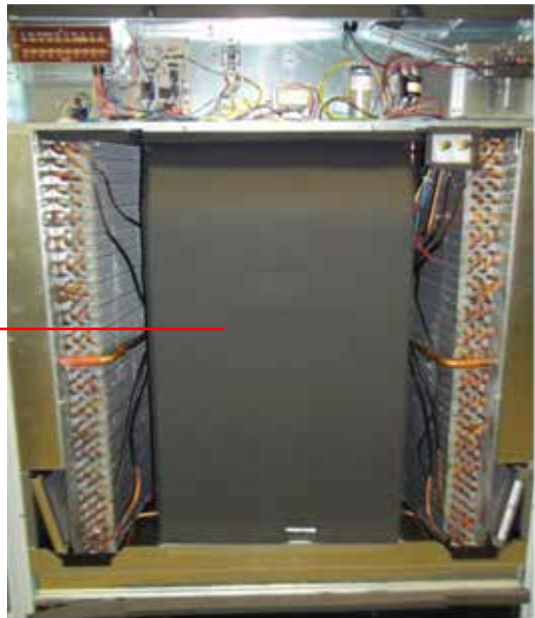
FIGURE 6 REMOVAL OF AIR DUCT
