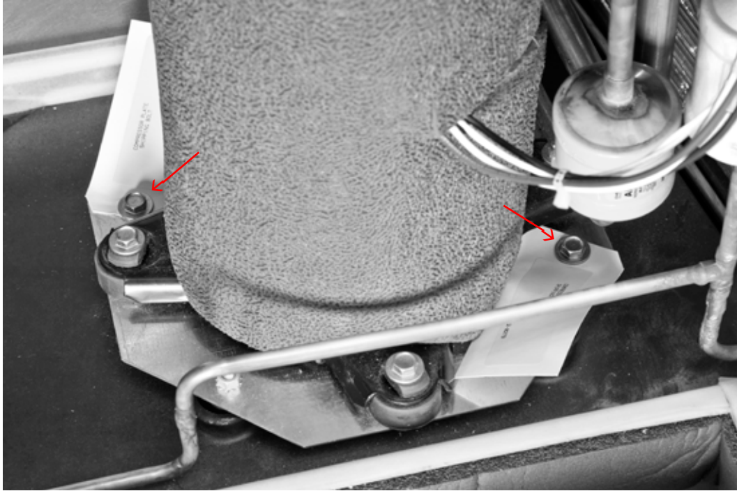
FIGURE 5 COMPRESSOR SHIPPING BOLTS
