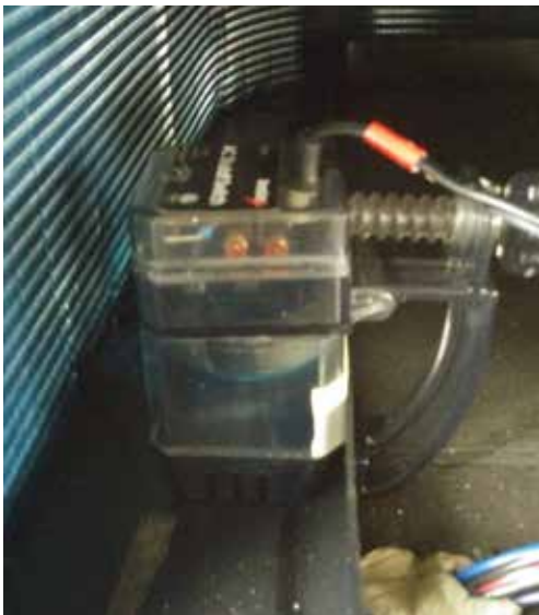
FIGURE 31 Outdoor Condensate Sensor
