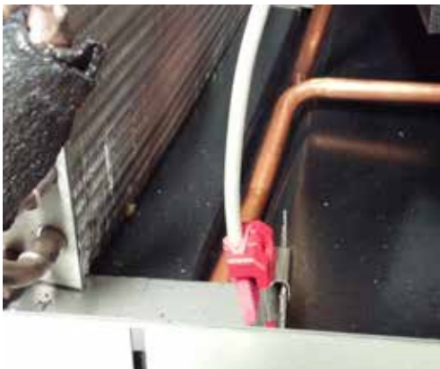
FIGURE 31 Outdoor Condensate Sensor
