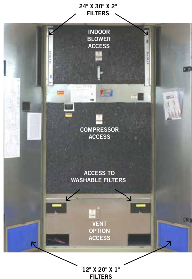
FIGURE 9 Filter Location
