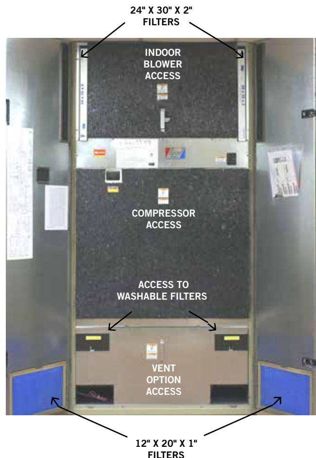
FIGURE 9 Filter Location
