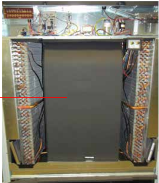
FIGURE 6 Removal of Air Duct
