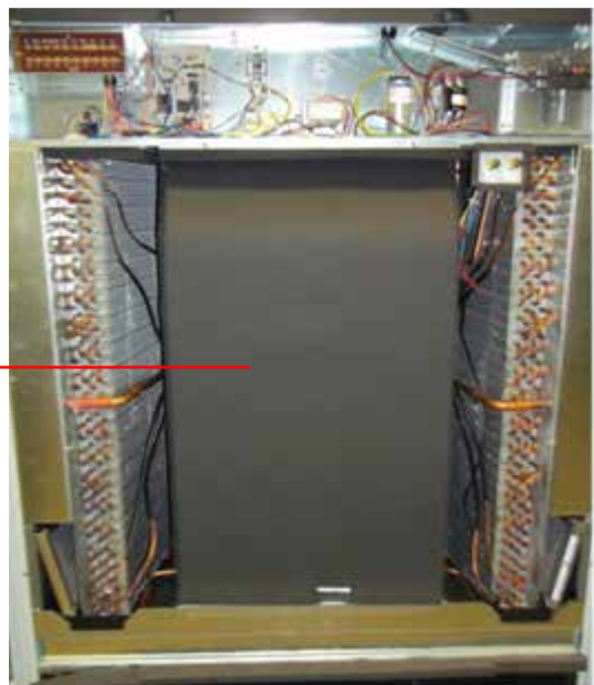
FIGURE 6 Removal of Air Duct
