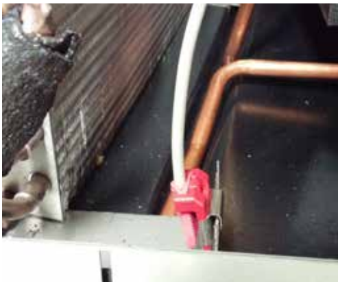
FIGURE 35 Outdoor Condensate Sensor
