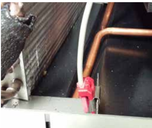
FIGURE 35 Outdoor Condensate Sensor
