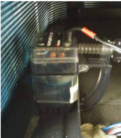
FIGURE 35 Outdoor Condensate Sensor
