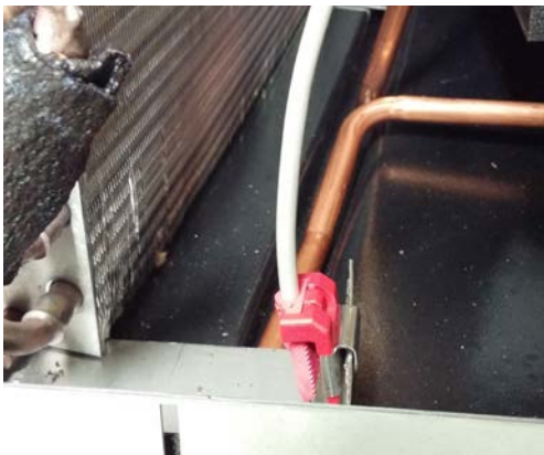
FIGURE 35 Outdoor Condensate Sensor
