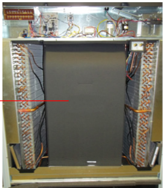
FIGURE 6 Removal of Air Duct
