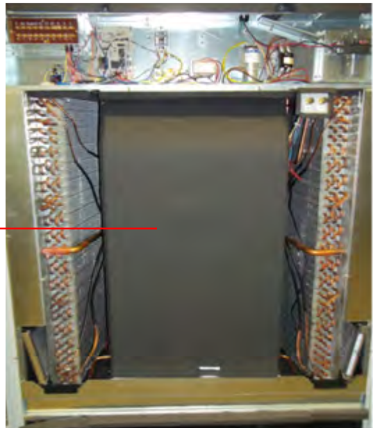
FIGURE 4 REMOVAL OF AIR DUCT
