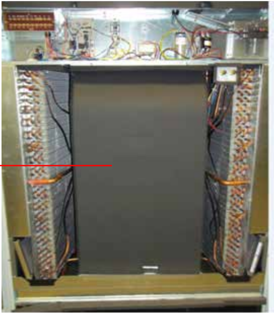
FIGURE 4 REMOVAL OF AIR DUCT
