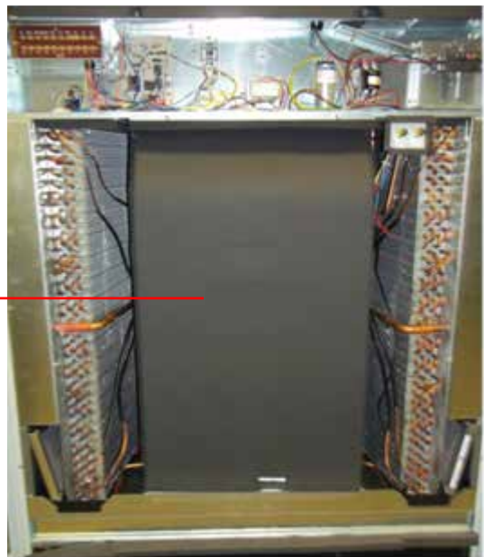
FIGURE 4 Removal of Air Duct
