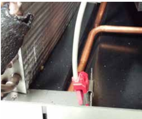
FIGURE 19 Outdoor Condensate Sensor
