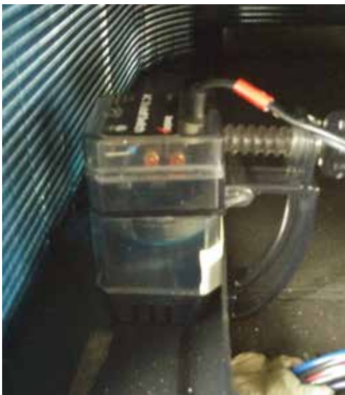
FIGURE 19 Outdoor Condensate Sensor
