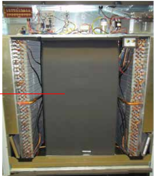
FIGURE 4 Removal of Air Duct
