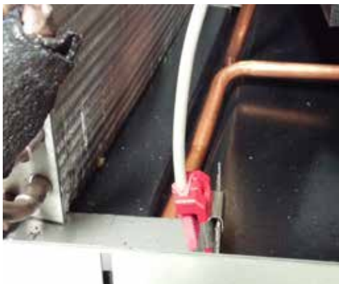
FIGURE 19 Outdoor Condensate Sensor
