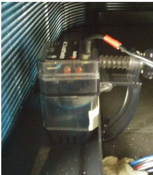
FIGURE 19 Outdoor Condensate Sensor
