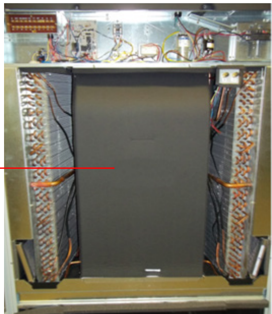
FIGURE 4 Removal of Air Duct
