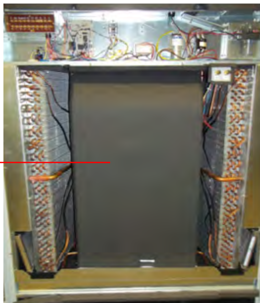
FIGURE 6 REMOVAL OF AIR DUCT
