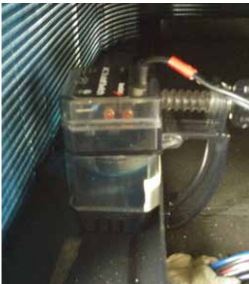
FIGURE 27 OUTDOOR CONDENSATE SENSOR
