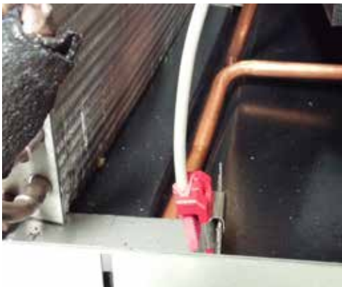
FIGURE 27 OUTDOOR CONDENSATE SENSOR
