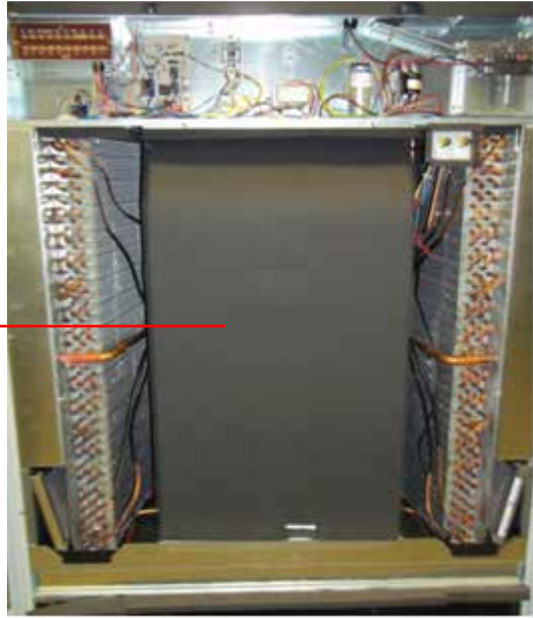
FIGURE 5 REMOVAL OF AIR DUCT
