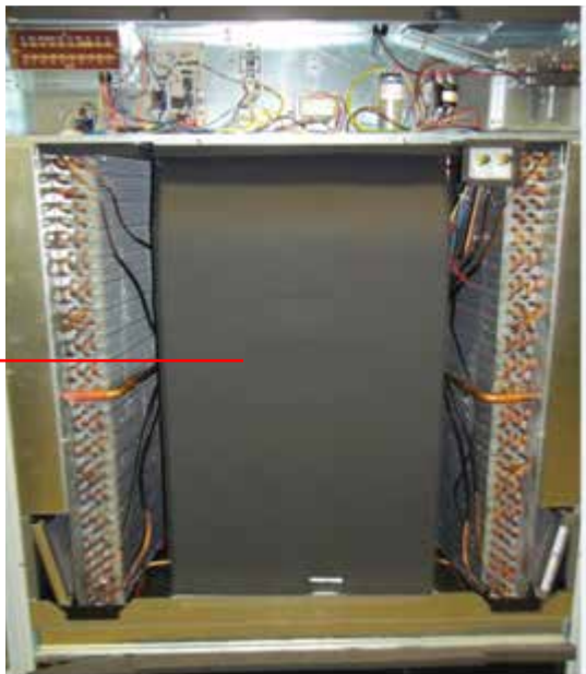
FIGURE 5 Removal of Air Duct
