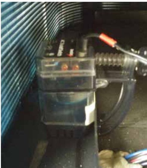
FIGURE 34 Outdoor Condensate Sensor
