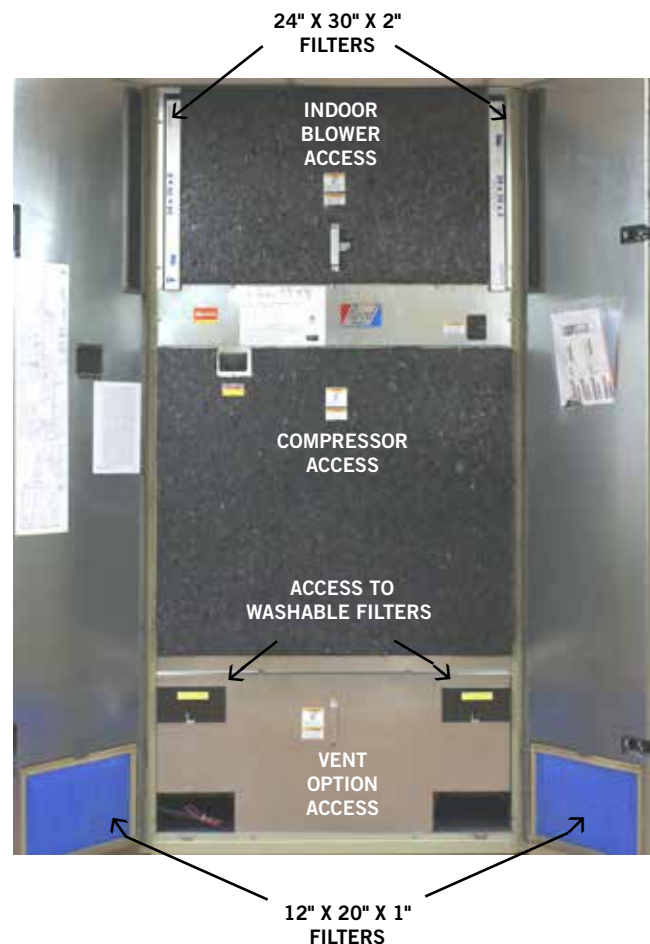
FIGURE 9 Filter Location
