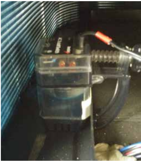
FIGURE 34 Outdoor Condensate Sensor
