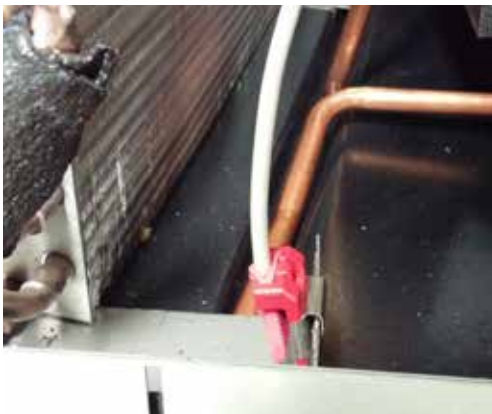
FIGURE 34 Outdoor Condensate Sensor
