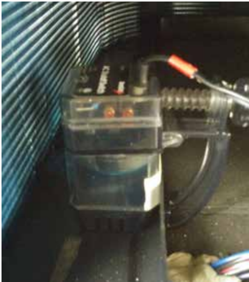
FIGURE 35 Outdoor Condensate Sensor
