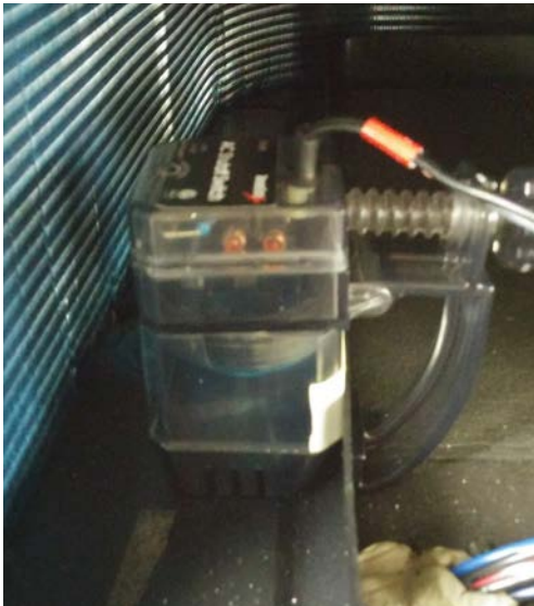
FIGURE 35 Outdoor Condensate Sensor
