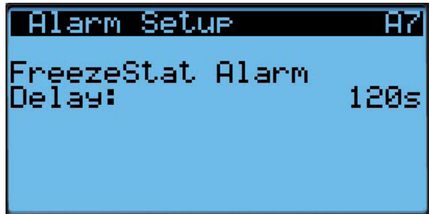
FIGURE 21 Adjusting Freezestat Alarm Delay
