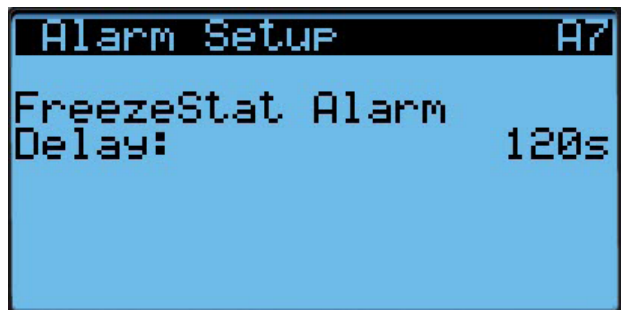
FIGURE 22 Adjusting Freezestat Alarm Delay
