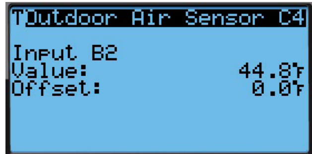
FIGURE 51 Outdoor Air Sensor
