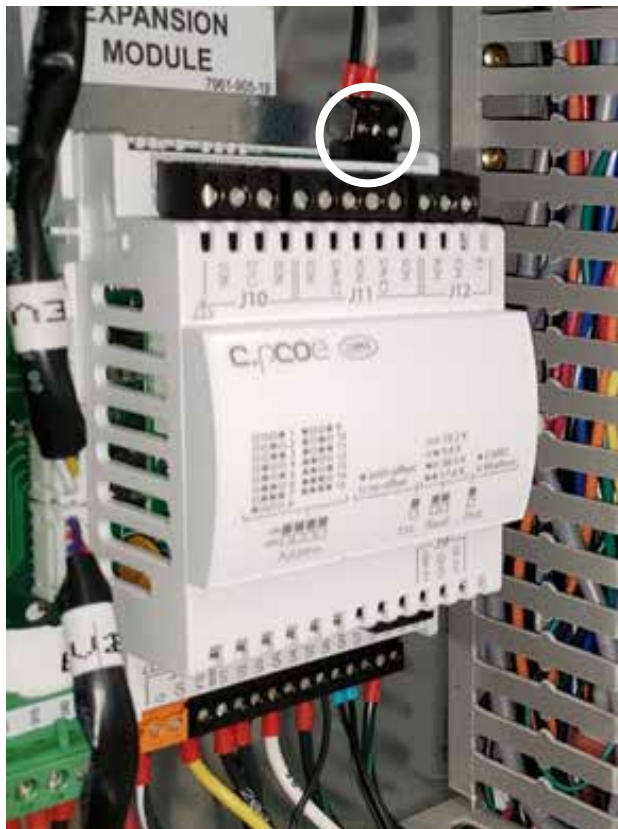
FIGURE 61 Unplug Modbus from Expansion Module
