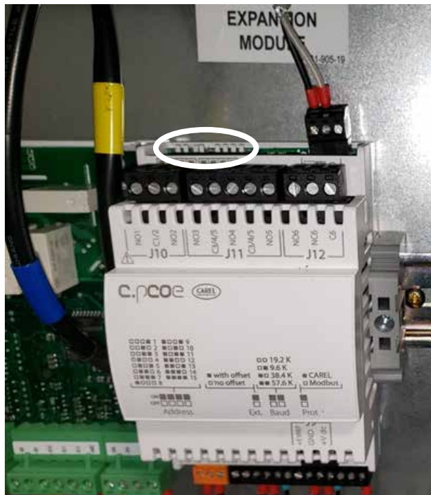
FIGURE 79 DIP Switch Location
