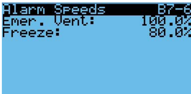
FIGURE 29 Adjusting Emergency Vent and Freeze Speeds
