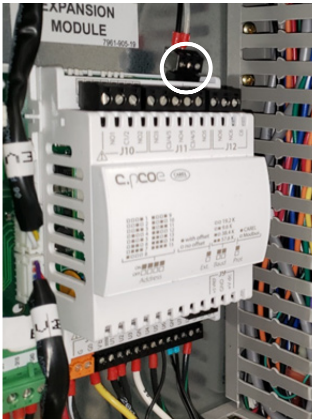
FIGURE 88 Unplug Modbus from Expansion Module
