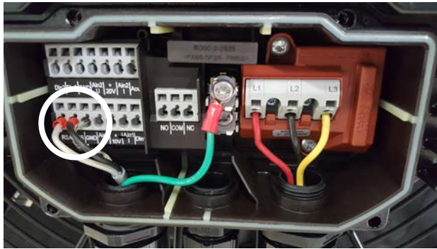
FIGURE 88 Unplug Modbus from Expansion Module
