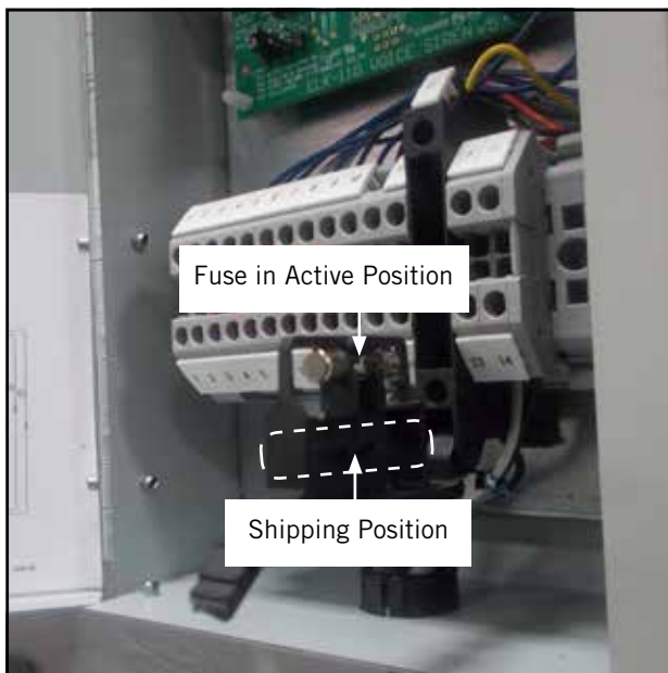
FIGURE 1 BG1000 Fused Power Supply Terminal
